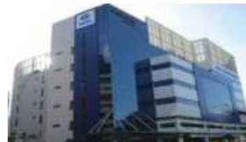
● Tata Communications Exchange
