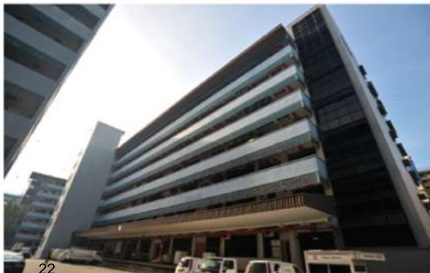
Toa Payoh North 1 Cluster before redevelopment
